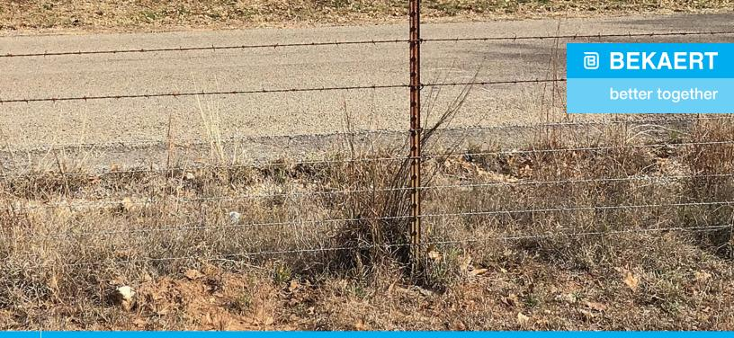
Texas rancher, Don Casey only uses high-tensile wire with a protective coating. Forty years ago he tested low-carbon, noncoated wire and Bekaert's high-tensile barbed wire on a fence along Blanco County Road 302. The results speak for themselves.
