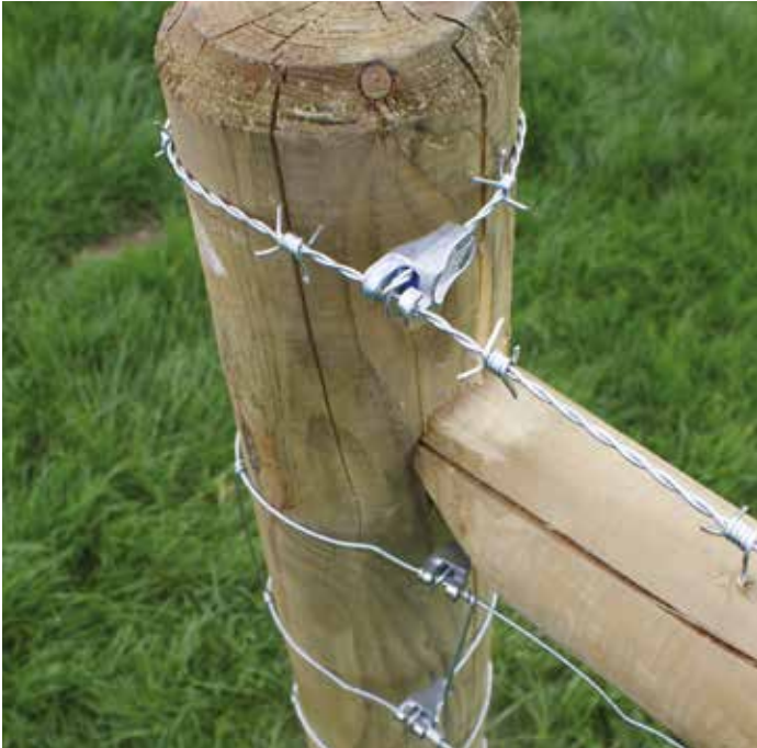
T-Clip 2 - Used to terminate barbed wire..
