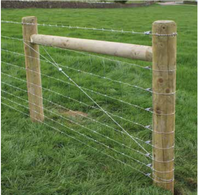
GPAK 4 - Bracing the end of a fencing run
