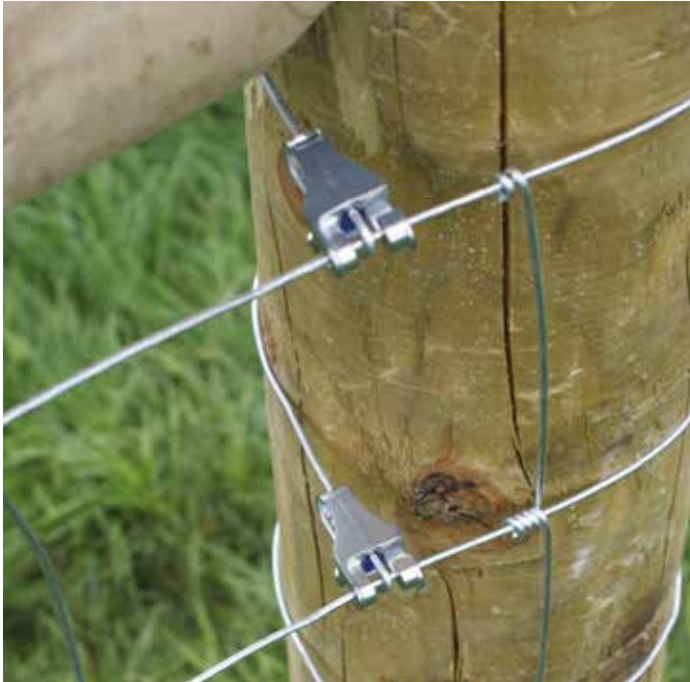
T-Clip 1 - Installed on a stock fence.
